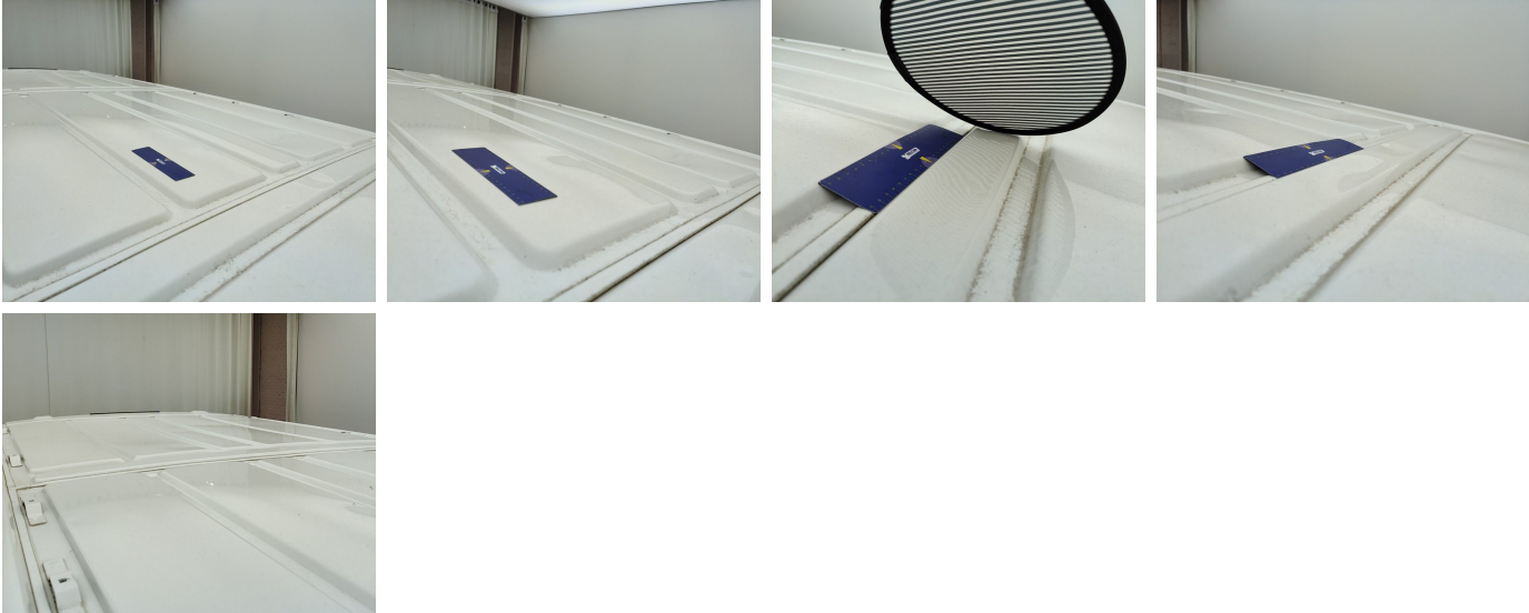
Roof // Repair & Painting-dent
