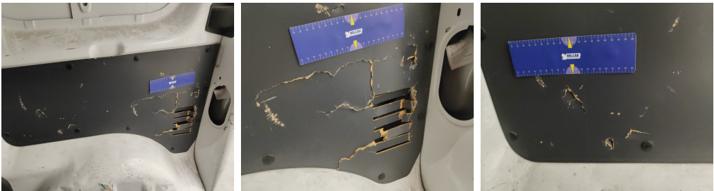
Interior // Repair 2-cracked
