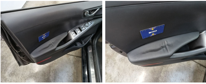
Front Left Door Interior Coating // Replace Completely-scratch + dent
