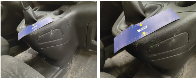
Central Console // Repair-stain
