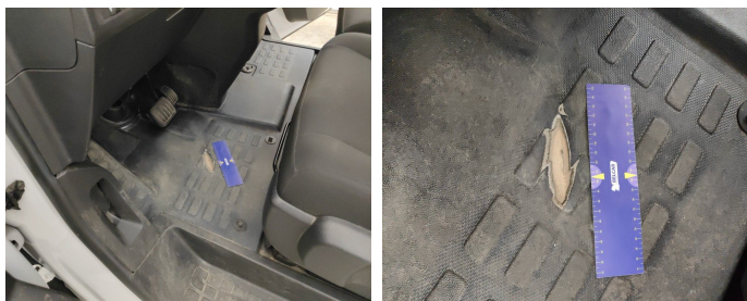
Interior // Repair 1-hole
